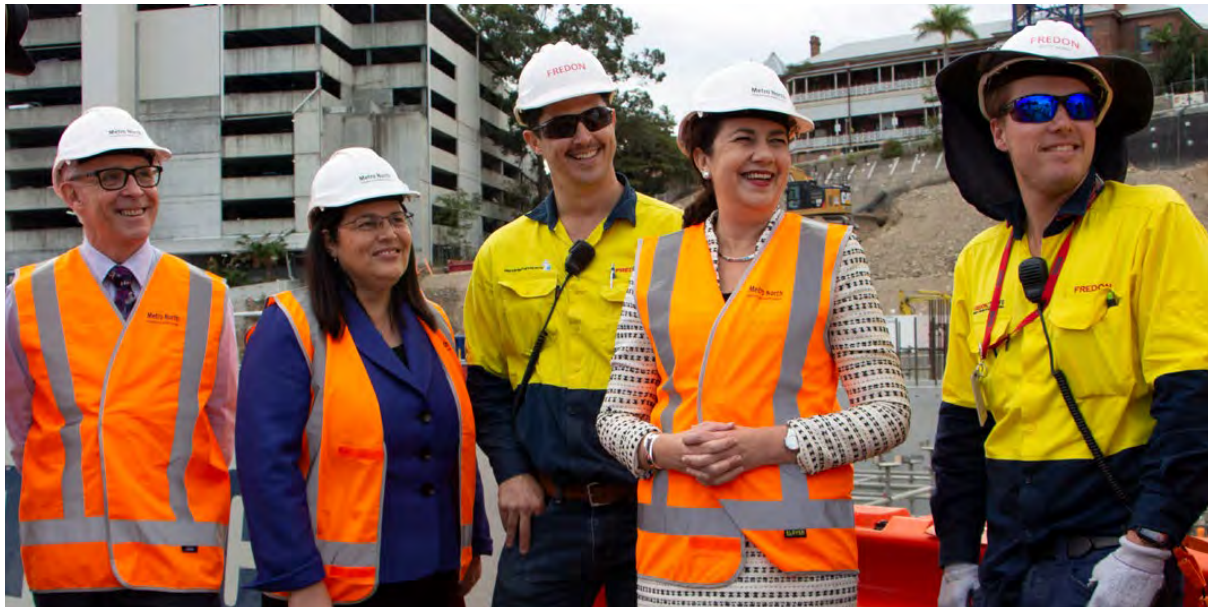
Premier Annastacia Palaszczuk, Member for McConnell Grace MP and Metro North Hospital and Health Board member Geoff Hardy inspecting works on the site of the $340 million specialist public health facility.
