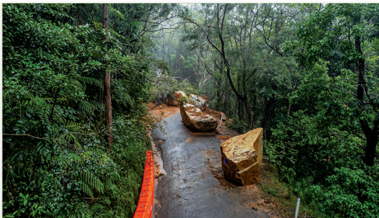
Impacts from the Far North Tropical Low: boulders on Mount Spec Road, Nywaigi Country—Department of Transport and Main Roads.
