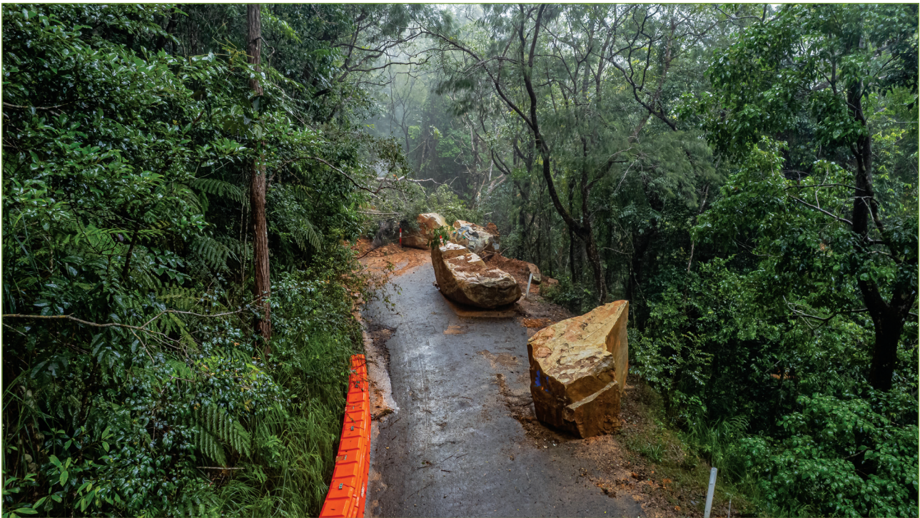
Landslide on Mount Spec Road, Nywaigi Country— Supplied: Department of Transport and Main Roads
