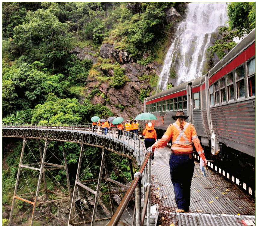
Inspecting landslide stabilisation works on the Kuranda Railway following extreme rainfall events, Djabugay Country— Wet Tropics Images
