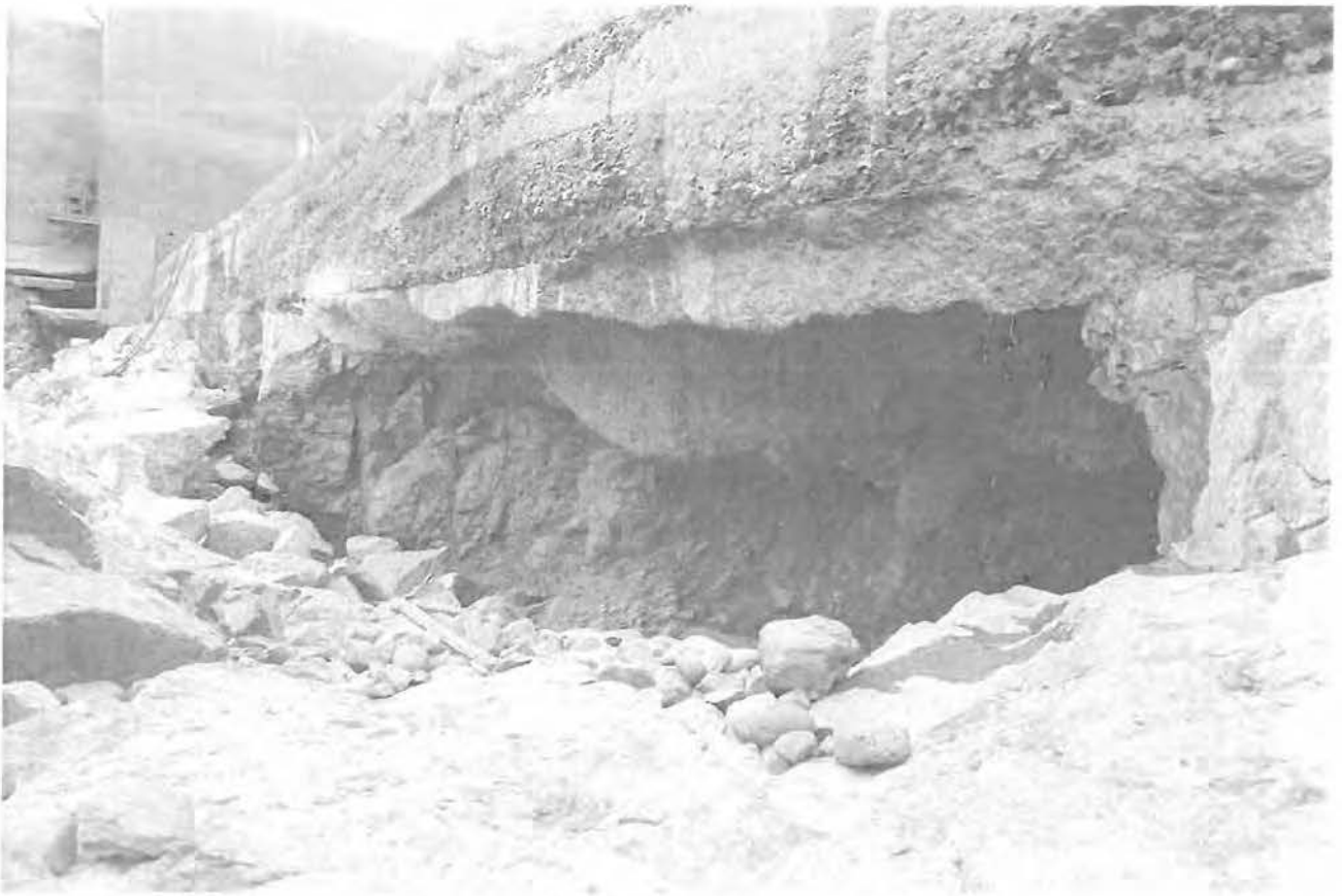
Damage to the wall of Paradise Dam, near Bundaberg, from flooding in 2013. (ABC News)
