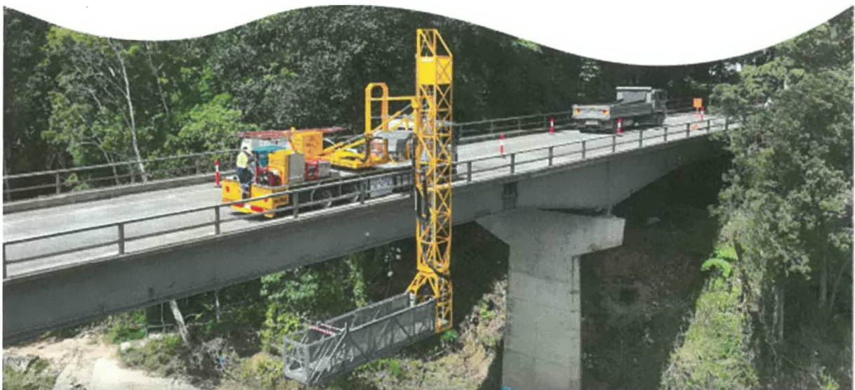
Image: An underbridge inspection unit in use as part of the SRMP. Source: TMR.
