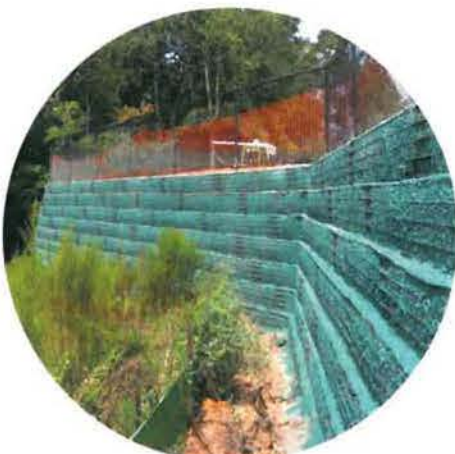
FLEXTERRA HYDRO MULCH & SEED APPLICATION TO GABIONS
