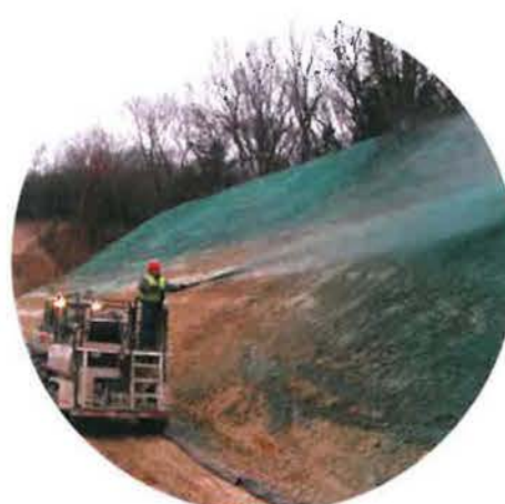
FLEXTERRA HYDROMULCH TO 1:2 BATTERS
