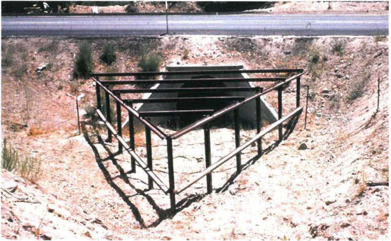
Figure 7. Example of inlet steel rail debris deflector (Source: HEC-9, Debris Control Structures)
