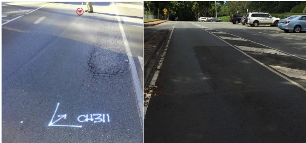
Figure 2G Restoring sealed road condition
