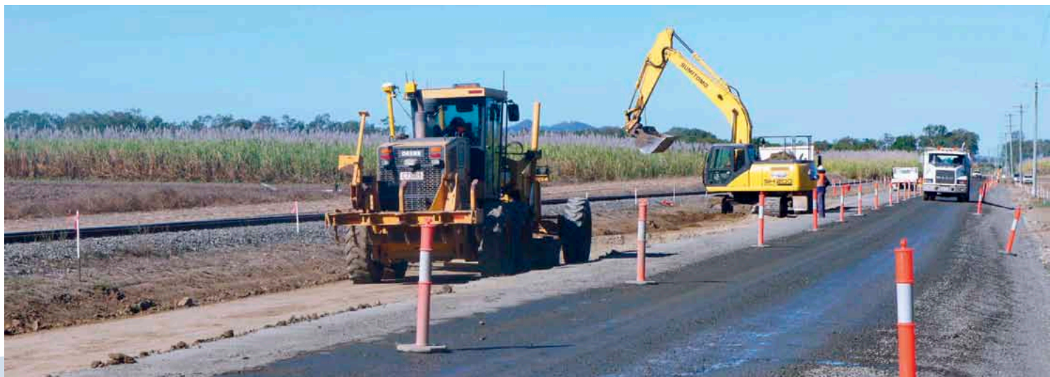
Subgrade treatment on Miran–Eton Road in the Mackay/Whitsunday region as part of the Transport Network Reconstruction Program
