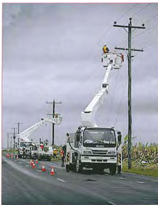
Cyclone-damaged powerlines under repair.
