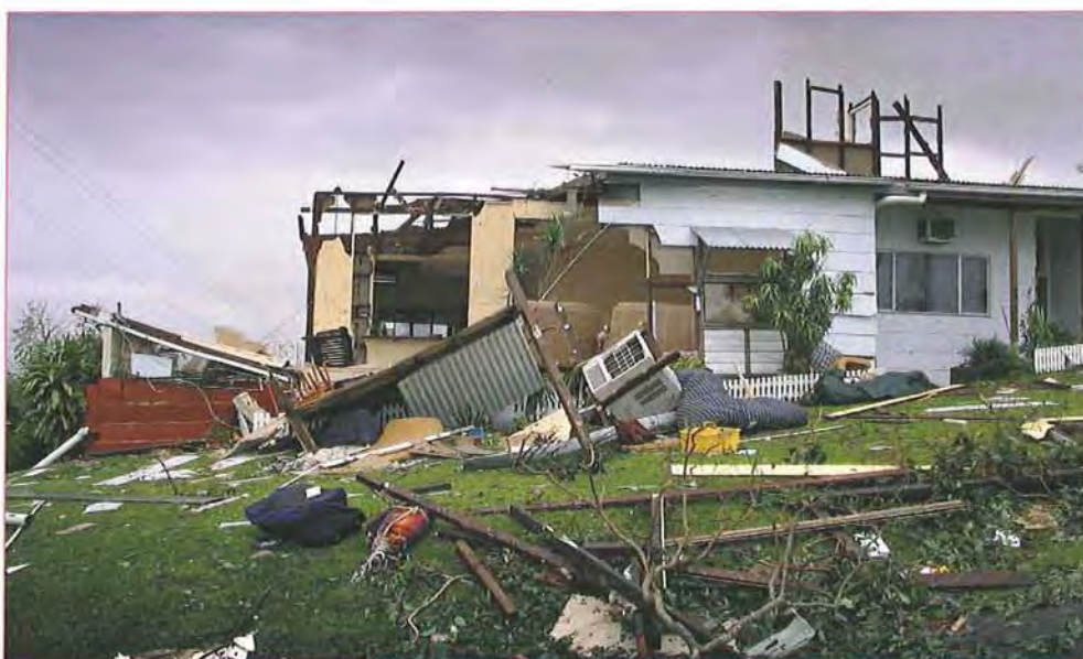
This picture shows the exposed construction materials in a cyclone-damaged building - relevant to the asbestos risk of recovery workers.
