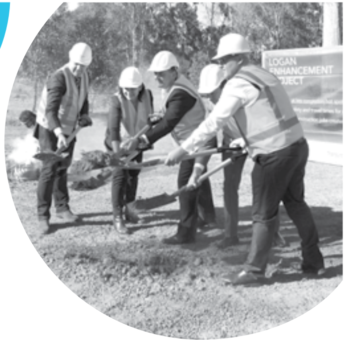
Above: Treasurer Curtis Pitt joined Linus Power MP, Leeanne Enoch MP, Logan Mayor Luke Smith, and Transurban Queensland Group General Manager Wesley Ballantine at a sod turning event to mark the start of construction for the Logan Motorway Enhancement project.
