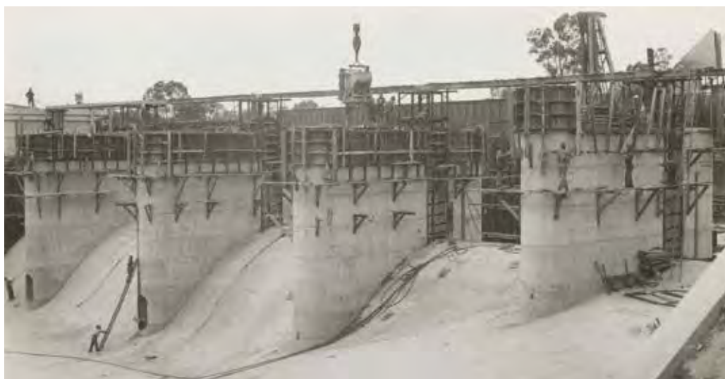
Construction of Yarrawonga Weir in 1938 (MDBA historic images collection)
