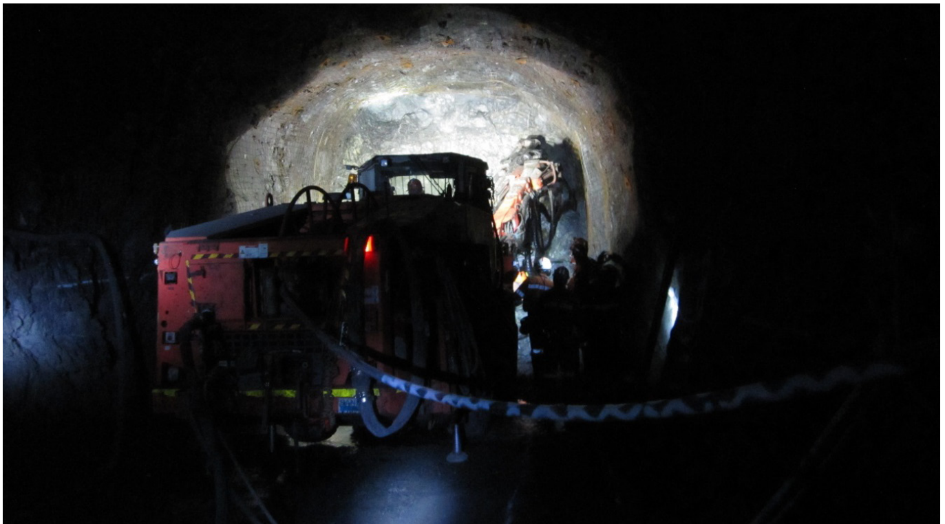
Twin boom development jumbo drilling out a face for charging Photo: DNRM
