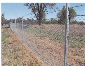
Track maintenance grading was carried out along approximately 248 kilometres of the fence. Drain clearing and vegetation slashing has been carried out where possible and herbicide spraying has assisted to control vegetation regrowth on both sides of the fence.
