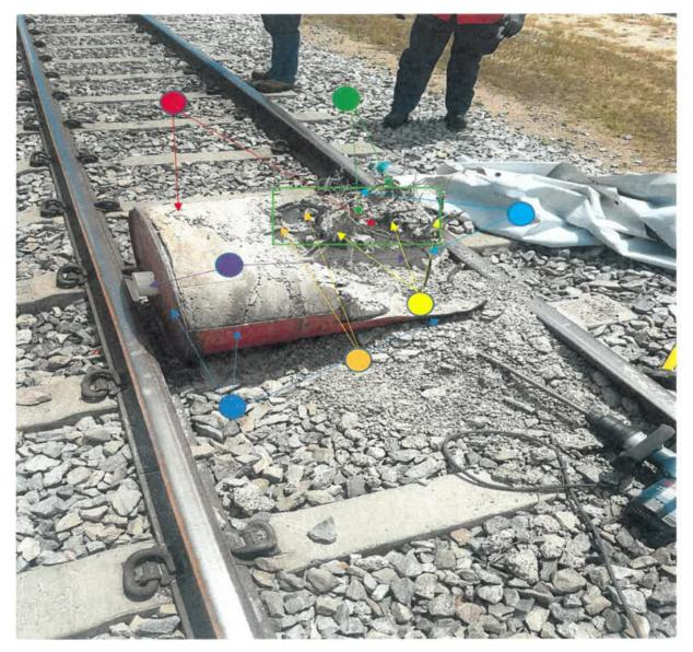
Exhibit F shows the exposed contents of a 'Dragons Den' being a 44 Gallon drum. Visible from the photograph as a part of the contents. It appears that the top / bottom of the drum and a section of the side has been removed the first of the contents been exposed through excavation of the sand and gravel
