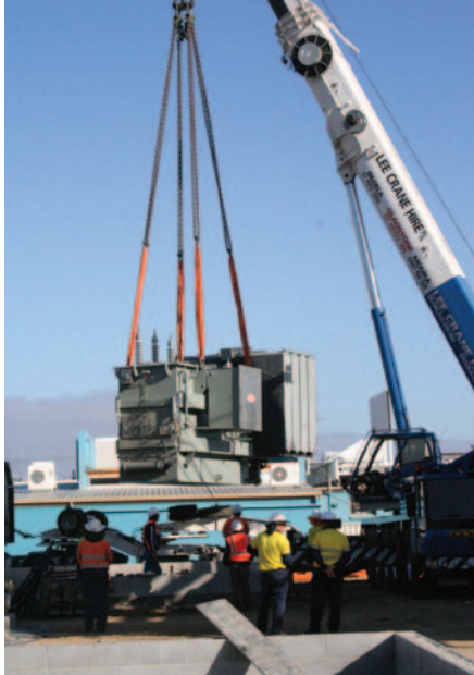
Work is well advanced on the new $26 million Berserker zone substation that will boost electricity supply to the rapidly growing North Rockhampton area, with civil works commencing in March and the 50 tonne transformers now lifted into position.
