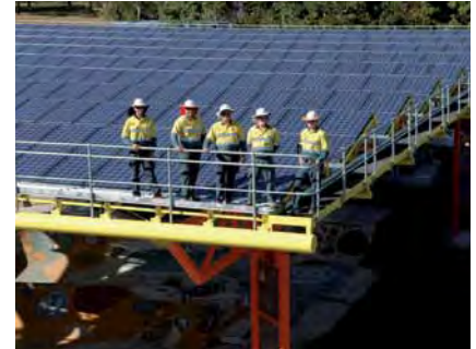
The Magnetic Island Solar Skate Park's 100kW photovoltaic system was commissioned this year. As well as being the largest solar array in Queensland, it will provide solar shade for skate park users, a family barbecue and picnic pavilion, a sporting team visitors pavilion and a stage for community presentations.
