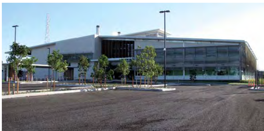
The new $26 million complex in Mackay will bring the benefits of a centralised presence to the Mackay region. It features an eco-link space incorporating natural lighting and a combination of air conditioning and natural ventilation to provide an open-plan meeting area to help foster the cross-workgroup relations central to a high performance culture.
